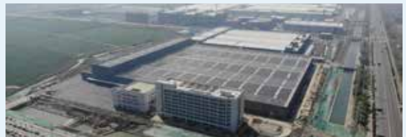
Changzhou New Energy Zero-Carbon Pilot Factory
