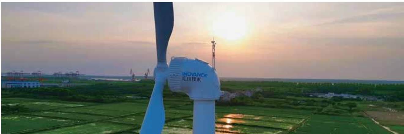
Wind Turbine at Yueyang INOVANCE
